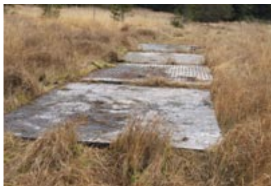
Fig. 107: Pontoon plates for increasing the bearing capacity of the terrain, Nové Údolí, November 2020 (I. Buřková)
