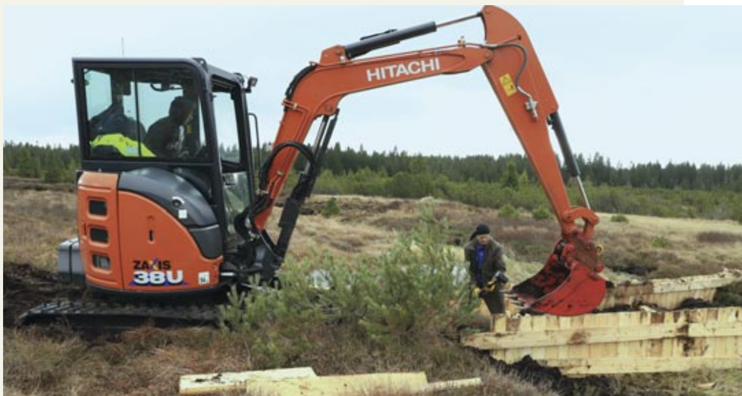
Fig. 256: Construction of dams made of hammered planks at the Jezerní slat site, November 2022 (I. Buřková)
