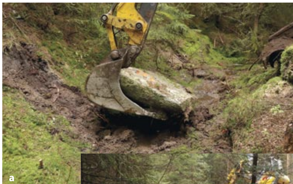
Fig. 138a, b, c: Placing large boulders, soil and sods into the erosion gully in the route of the original stream at the Gerlova Hut locality. Earthworks being implemented by the technique in September 2021 (a, b) and the situation in the third year after restoration in June 2024 (c). The bottom of the stream was raised by a total of 40-50 cm. (I. Buřková)
