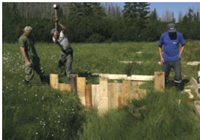
Fig. 62: Manual installation of a dam from vertical planks at the Blatenská slať location, July 2006 (I. Buřková)
