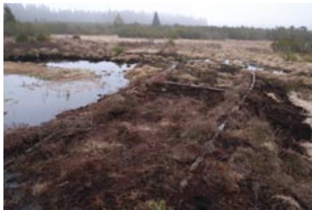
Fig. 102: An example of a massive double dam from planks with a large interspace filled with peat on Jezerní slat bog. The embankment of the dam is not sufficient considering the dimensions of the site, but it is functional. The water retained above the dam is re-directed into the peat bog on the left bank, February 2024 (I. Buřková)
