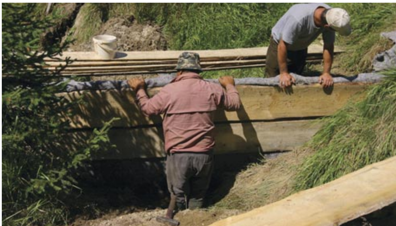
Fig. 60: The construction of a board dam in a prepared cut at the Rybárny – Javoří location, July 2008 (I. Buřková)
