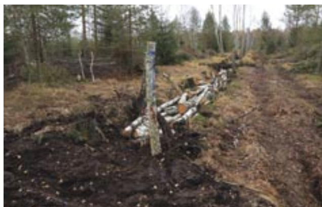
Fig. 77: Filling the space between dams in the blocked drainage channel using logs from prunings, Borková bog, October 2022 (I. Buřková)
