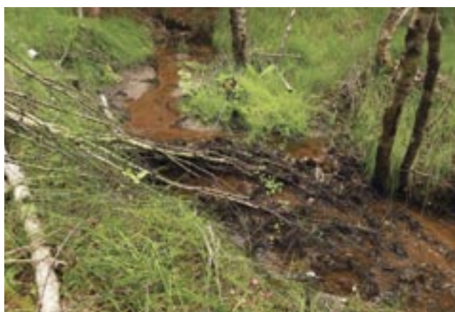
Fig. 148b: Simply laying birch from the bank prunings in a suitable direction into the small restored stream effectively promoted its riffling, sediment trapping and stabilization of the raised bed, Roviny site, July 2024 (I. Buřková)
