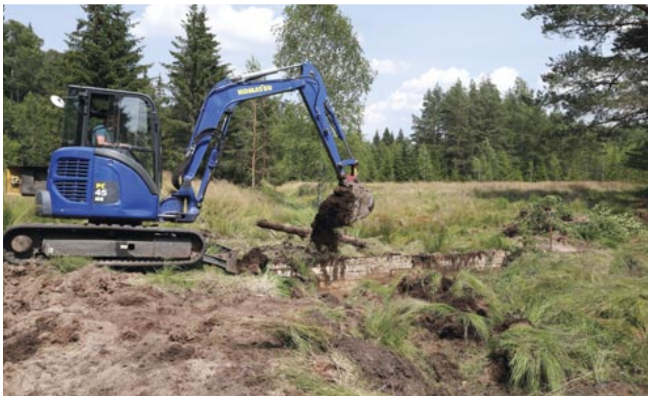
Fig. 74: Backfilling of dams with soil from bank mounds in the Raškov locality. The soil for backfilling should have a good consistency and adhesion. Clays are especially suitable, but also peat or moist loamy soil with only a small admixture of sandy fraction and stones (I. Buřková)
