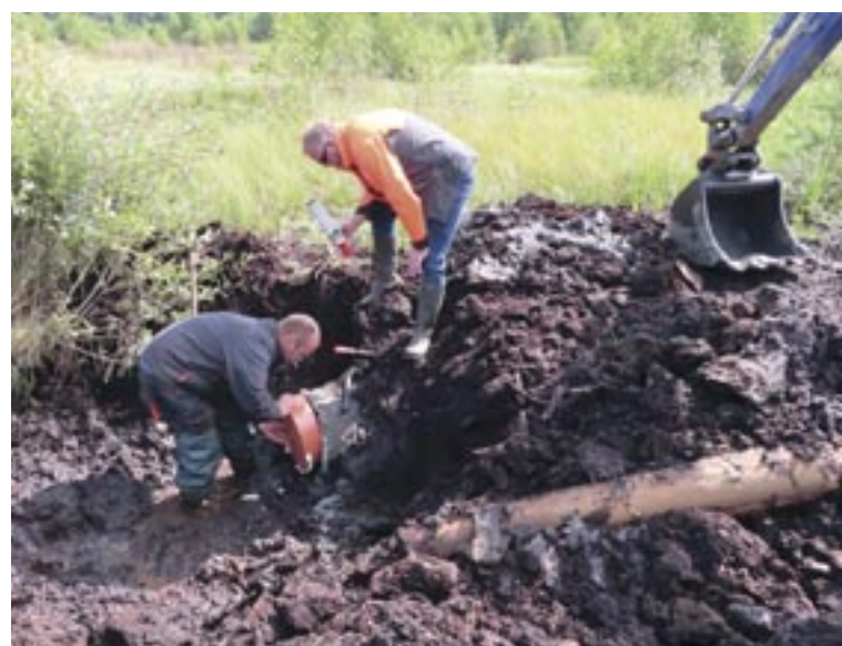
Fig. 83: Blinding of the remaining pipe segments with suitable plastic ends of the corresponding diameter on the mined Vlčí Jámy bog, August 2021 (E. Václavíková)
