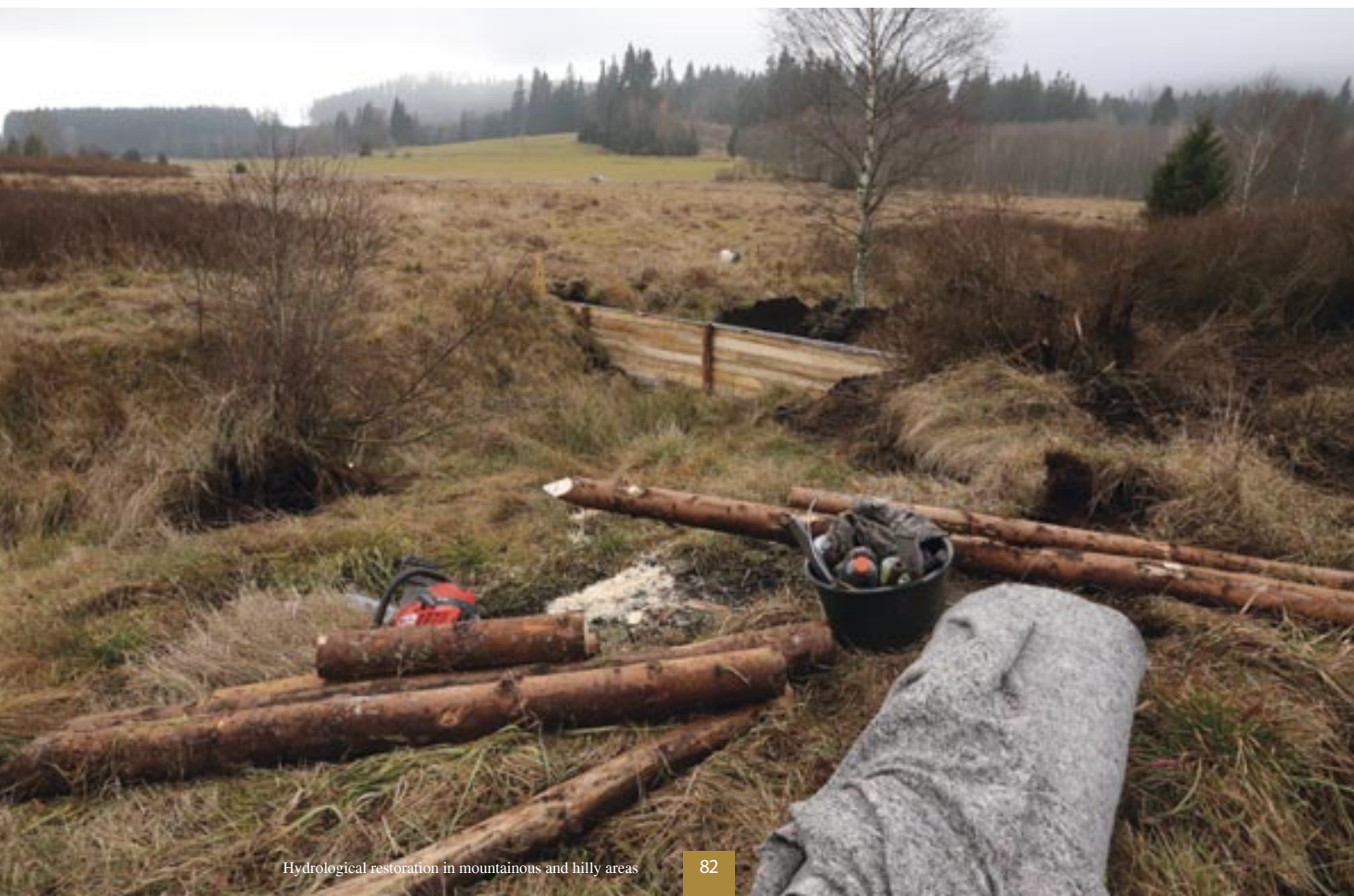
Fig. 98: Prepared geotextile and stabilization stakes, in the background a lately installed board dam in a deep channel at the site Dobrovodské louky. In this case, the logs were placed incorrectly and had to be delivered also to the air wall of the dam, November 2021 (I. Buřková)
