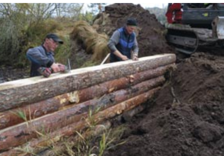
Fig. 143: During the construction of massive dams at the intersections of straight channels with the restored stream, logs cut on the upper and lower sides were used in a number of places, Kořenský stream, November 2023 (J. Zelenka)
