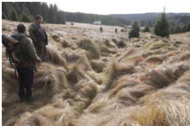
Fig. 75: Well-preserved and bulk embankments along the drainage channels are a welcome source of material for infilling the channels, Pod Skelnou location, April 2016 (I. Buřková)
