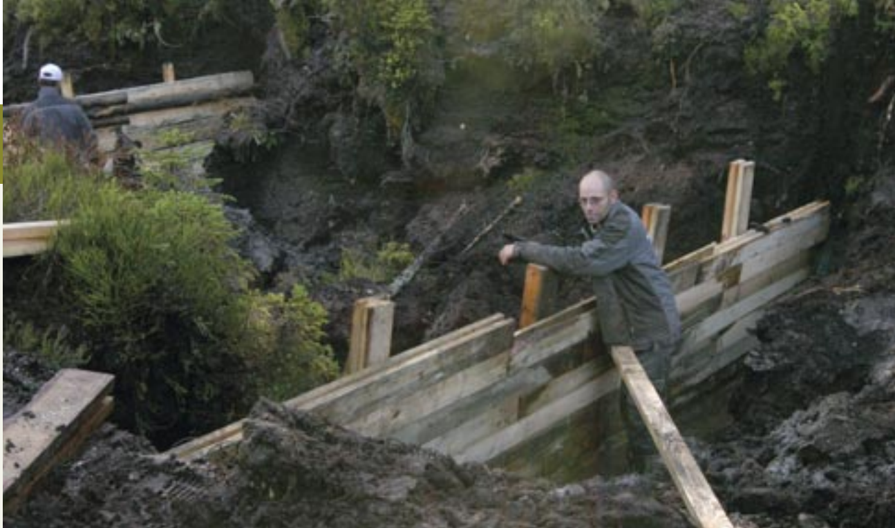
Fig. 278: Installation of the board walls in the erosion gully on the slopes above the Vltava River below Černohorský močál bog was technically very demanding, October 2014 (I. Buřková)
