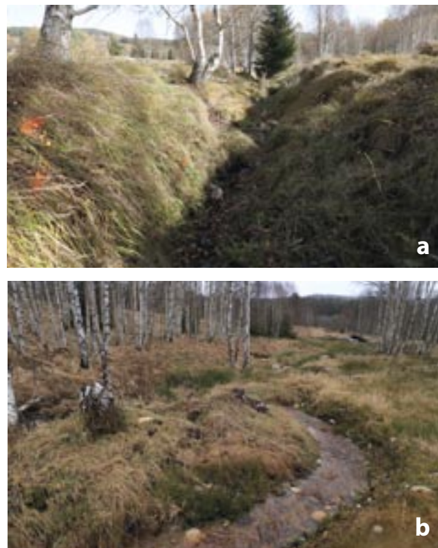
Fig. 141a, b: Restored natural stream bed directly in the line of straightened and modified watercourse 1 year after restoration, Pod Skelnou location, October 2021 (a) and January 2023 (b). The red marker in the foreground shows the level to which the bottom has been raised (I. Bufková)
