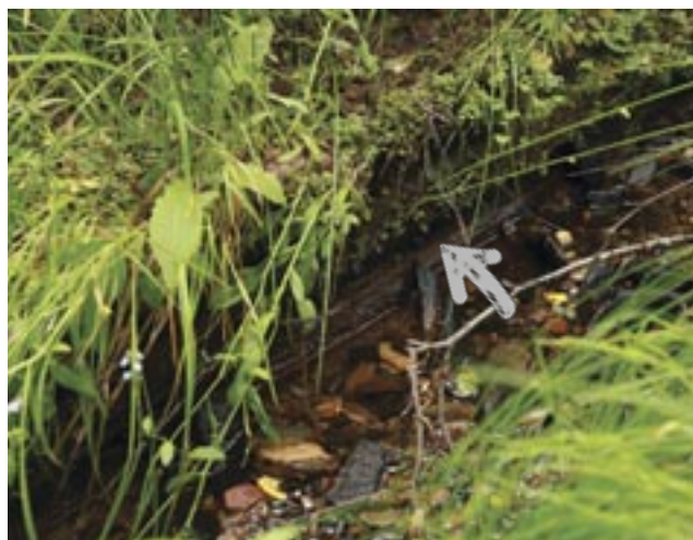
Fig. 151: The inconspicuous fortification of the banks in the small streams with longitudinally placed machined logs is often not visible under vegetation, but is very effective and must be removed, Zhůří, June 2024 (I. Buřková)
