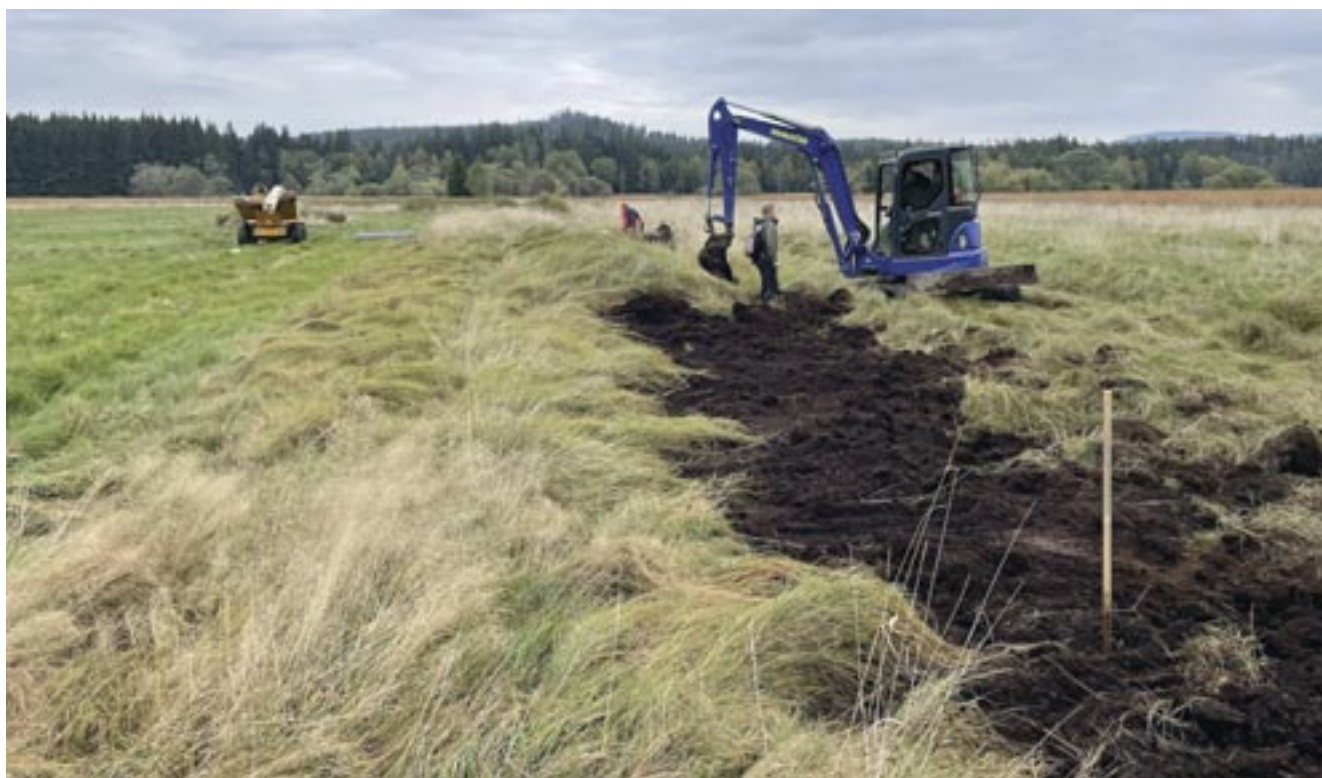
Fig. 286: Frequent inspections of the construction site and good communication with the contractor are a must for restoration projects. Disposal of the drainage channel in the Vltava floodplain at the Dobrovodské louky site, September 2021 (L. Linhart)
