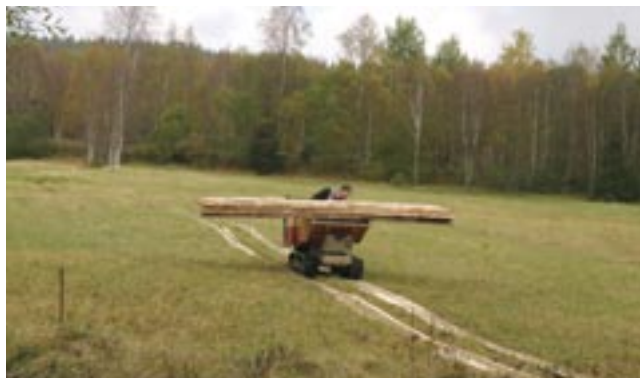
Fig. 69: An example of the use of a light dump truck to transport material on a sensitive surface. The use of planks made it possible to cross the peat meadow several times without signs of damage, Zhůří, I. stage, October 2014 (I. Bufková)
