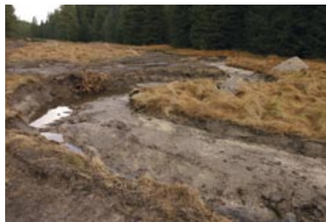
Fig. 144: Initiation piles of sand and gravel misplaced on the banks of the newly formed Hucina channel. The piles do not encroach into the channel and consist of too fine a fraction. Hucina, October 2013 (I. Buřková)
