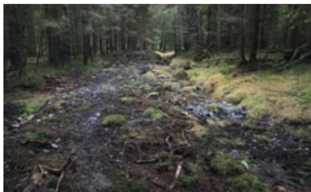
Fig. 78: Drainage channel blocked by a cascade of wooden dams and completely filled with soil, Devítka site, November 2020 (I. Buřková)
