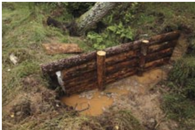
Fig. 101: Improperly constructed and inserted dam made of raw boards. The beveling of the board wall at the left bank and the failure of the side edge of the dam to reach the edge of the notch are evident, July 2020 (I. Buřková)
