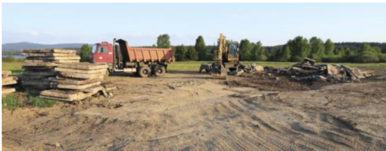
Fig. 122: Removal and disposal of firmed roads made of concrete panels that allowed the movement of technique during peat extraction is common part of the industrially mined bog restoration. Temporary deposition of panels intended for removal on the edge of the restored Borková peat bog, May 2023 (I. Buřková)
