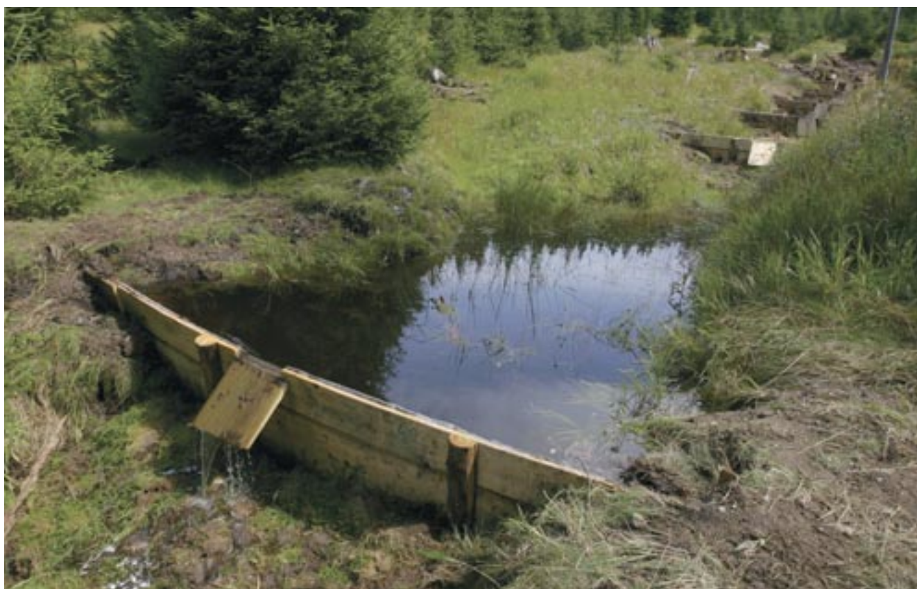
Fig. 103: In many respects, the damming was wrongly executed. The backfill is insufficient and the dam is not stabilized and protected. The spillway is too short, so the stream of water hits the bottom just below the dam, which it soon erodes and washes away. Such a measure is pointless, the cascade will break down over time and the function of the drainage channel will be re-established, project site Nad Rybárnou, August 2008 (I. Buřková)
