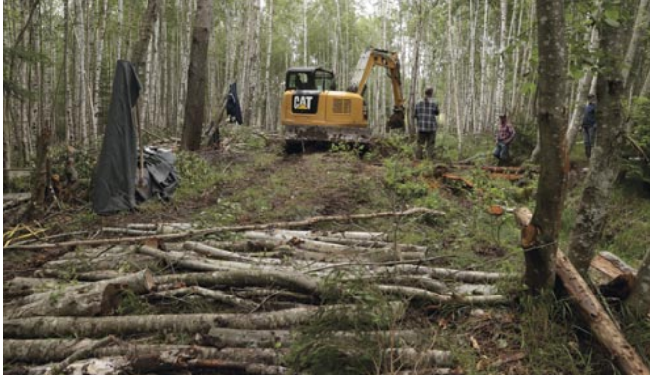
Fig. 71: Use of cut trunks to drive over wet parts with technique, Malý Bor, July 2020 (I. Buřková)
