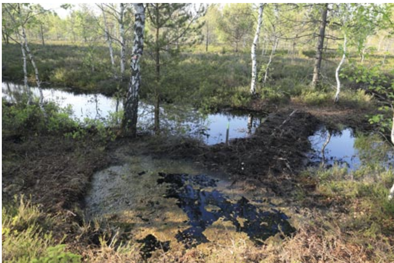
Fig. 118: Incorrect location of the depression made to obtain soil to fill the canal. The pool is too close to the edge of the dam backfill which could be easily bypassed by water flow and gradually washed out, May 2023 (I. Buřková)
