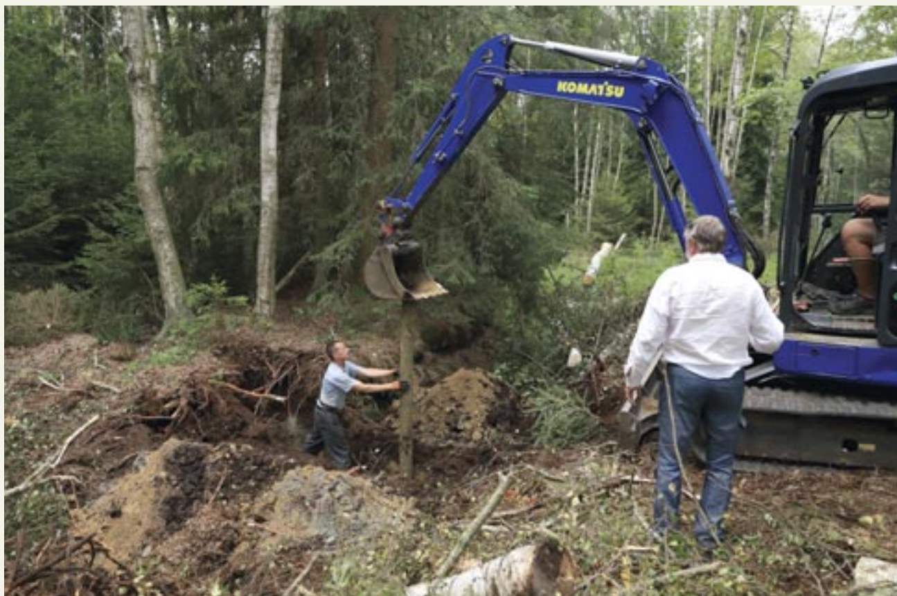
Fig. 239: Field work while blocking drainage channels in the Rovina site, August 2022 (I. Buřková)
