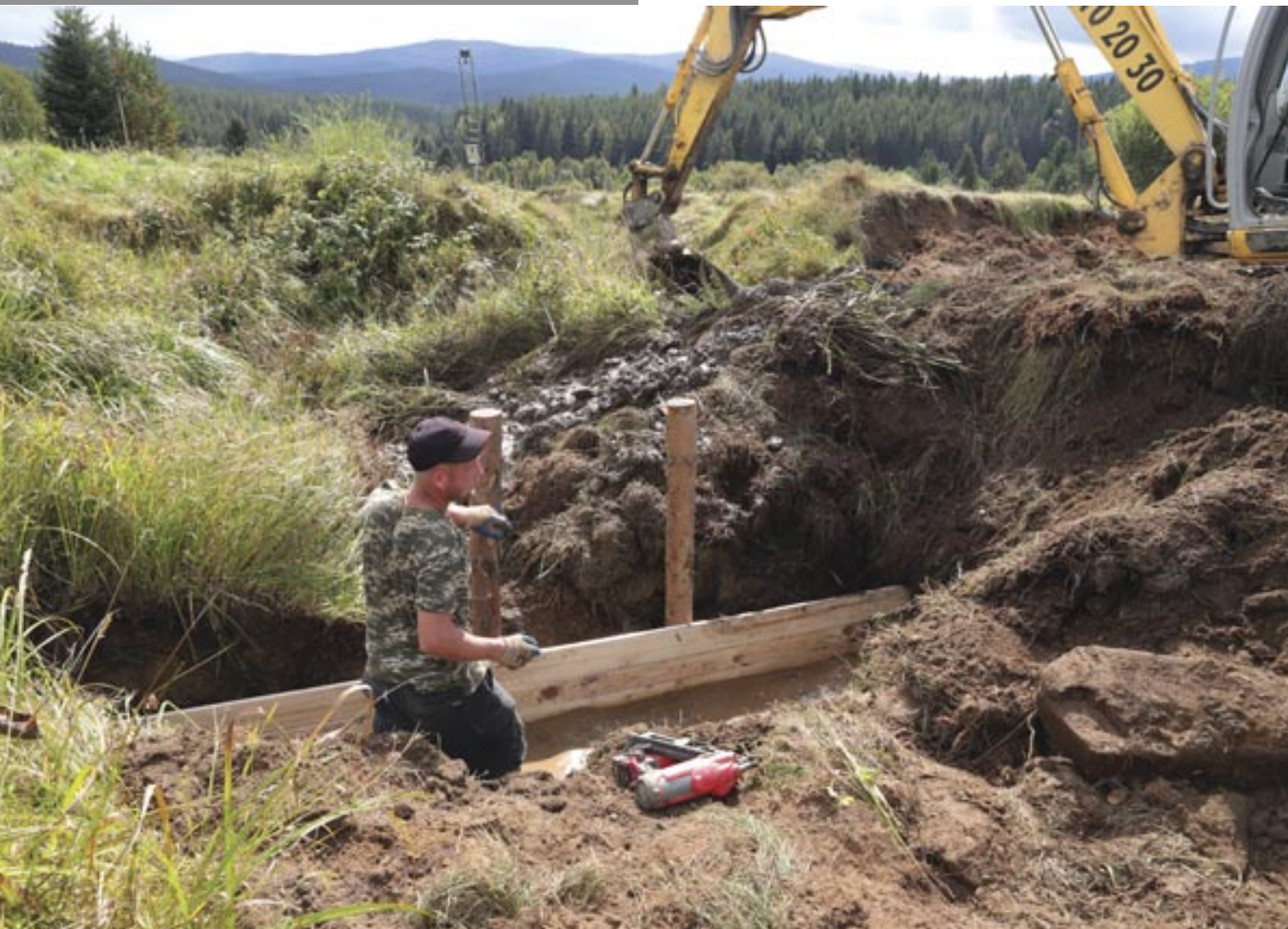
Fig. 287: Complete blocking of the drainage ditch before it is filled by soil at the Pod Skelnou site, September 2021 (I. Buřková)
