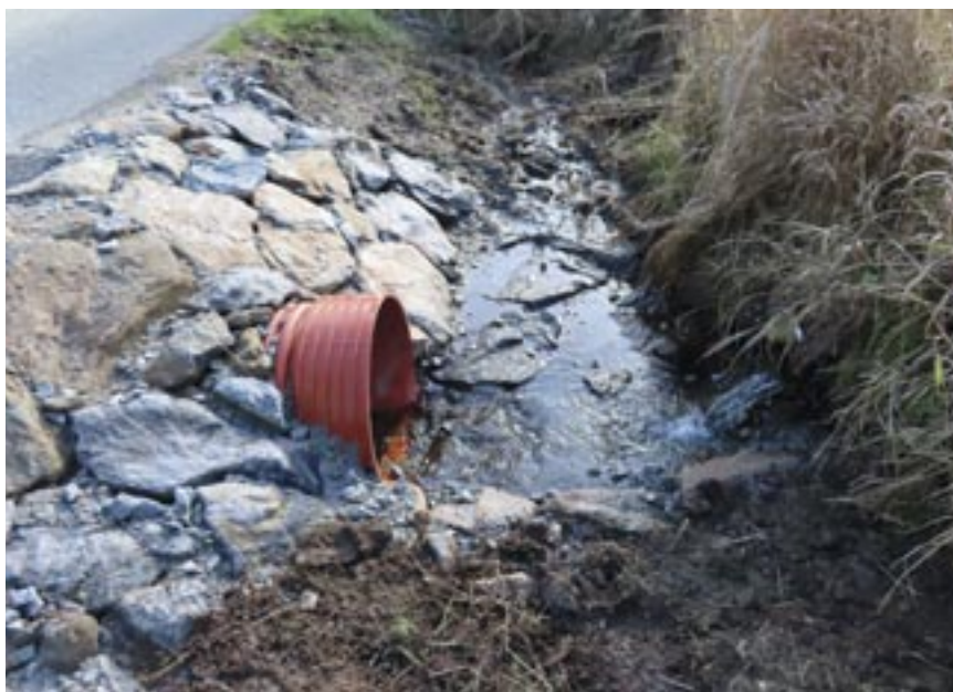
Fig. 86: New culverts installed in the construction of roads on slopes are also an important measure, as they will enable a more even transfer of water to the drying parts under the road, Novosvětské slatě, April 2022 (E. Václavíková)
