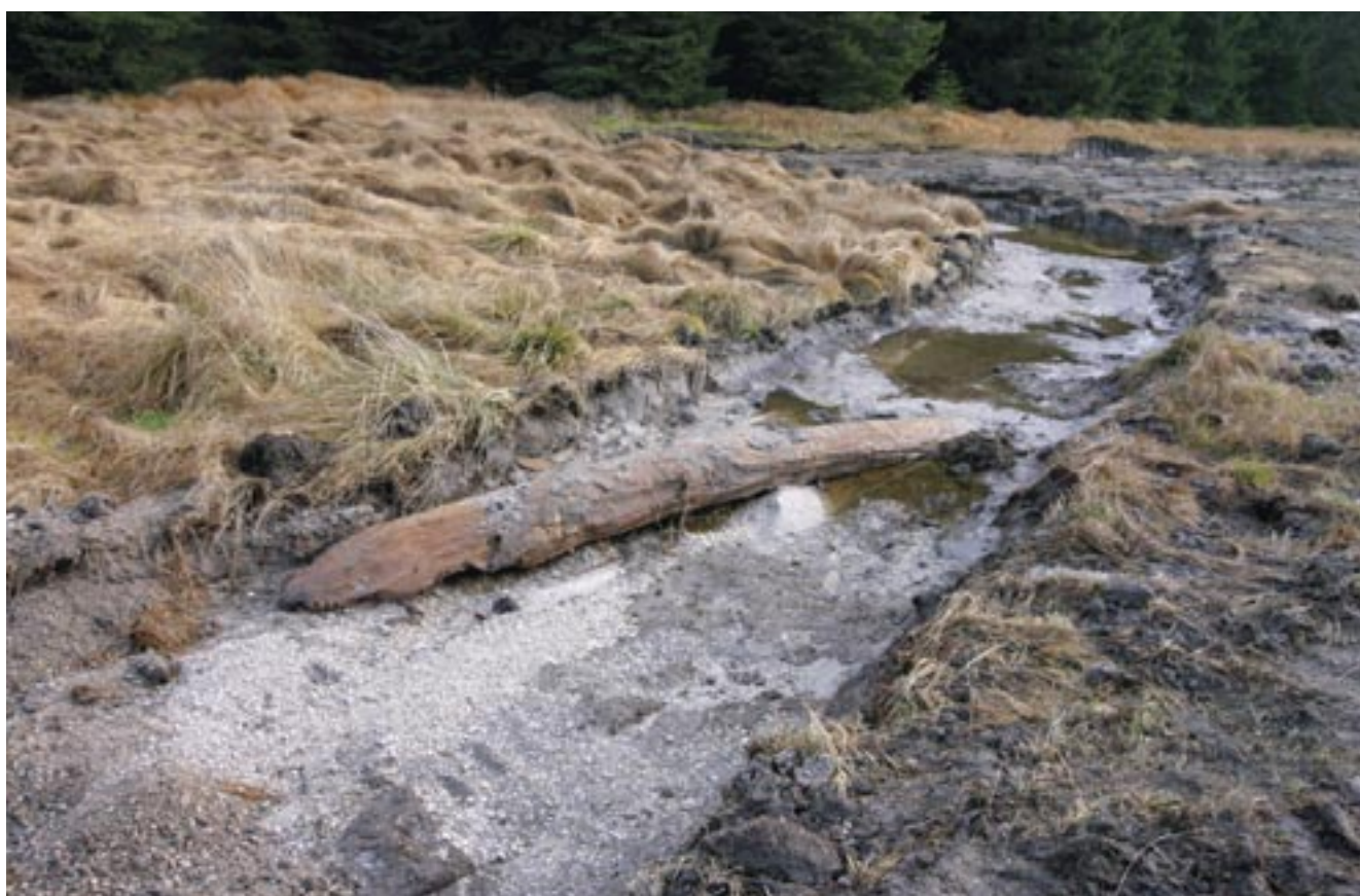
Fig. 153: Pieces of wood, stones and large boulders are an important element in the restored channel, Hucina, October 2013 (I. Buřková)
