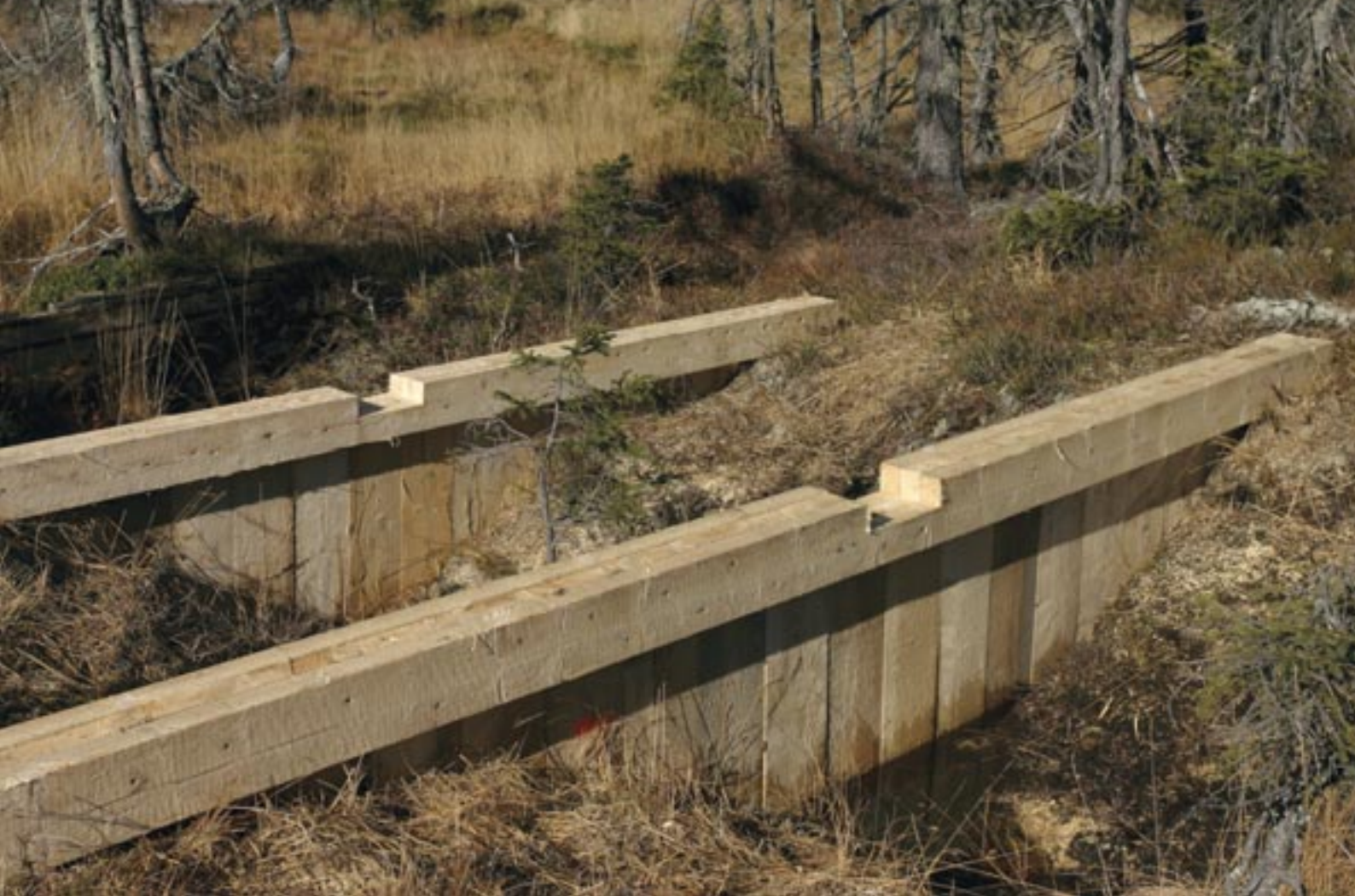
Fig. 99: Dams made of vertically hammered planks immediately after installation, before filling the channel with soil material and water. Luzenská slat', October 2005 (I. Buřková)
