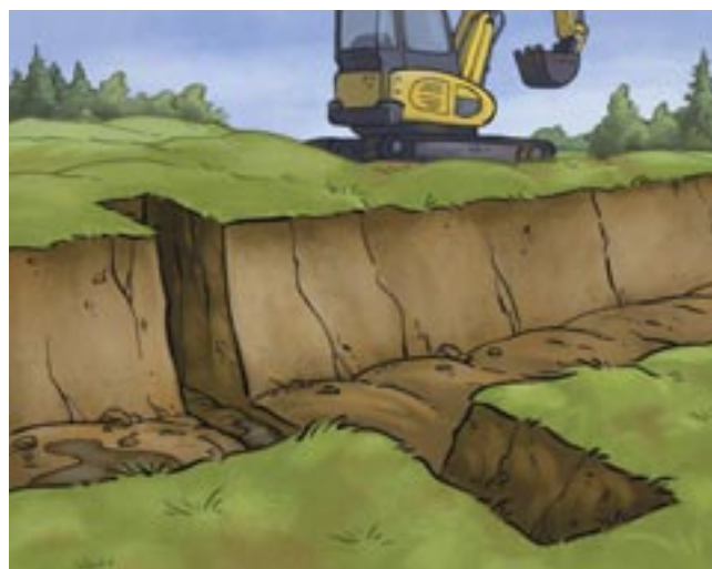
Fig. 58: Excavated cut for installation of the dam made of plank dam
