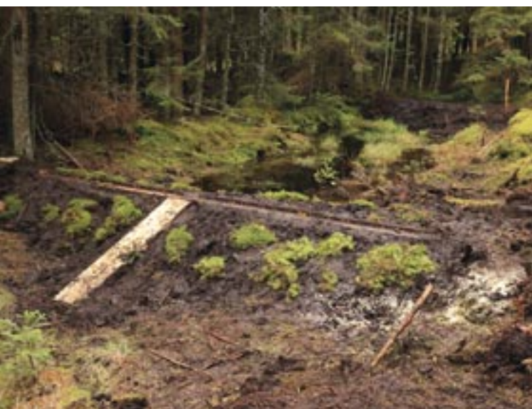
Fig. 61: A well-installed dam with an overflow in case of outflow during high water levels. Proper backfilling on the front air side of the partition and insufficient backfilling on the upper (water) side, Devítka location near village of Stožec, November 2020 (I. Buřková)
