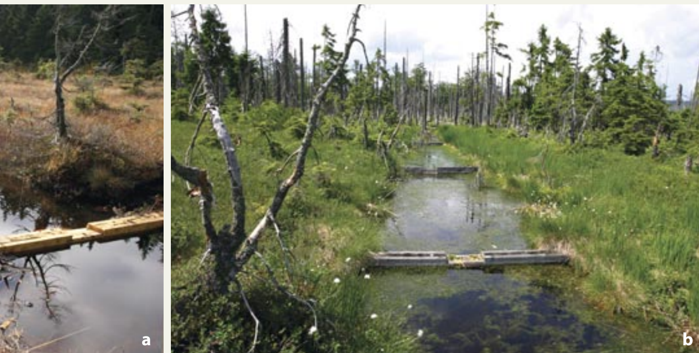
Fig. 273: The drainage channels at the Schachtenfilz site were manually dammed using woody dams without backfilling. Condition of the dams in October 2008 immediately after restoration (a) and ten years later in June 2018 (b) (I. Buřková)
