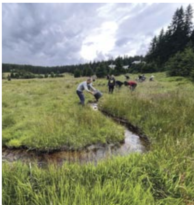
Fig. 145: Volunteers helping to fill in the missing rocky substrate in the stream section of the restored small stream at Rybárny I, July 2022 (L. Linhart)
