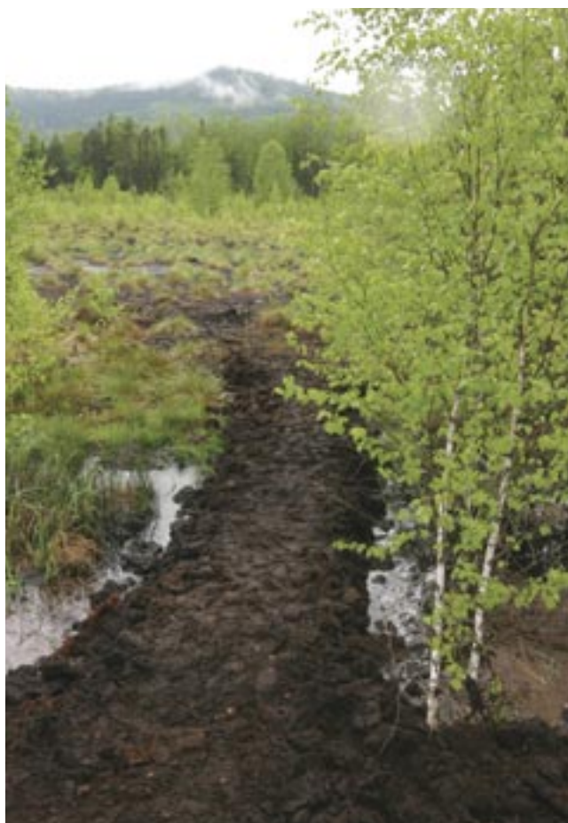
Fig. 73: The gravity dam created from compacted peat on Soumarský Most bog, June 2012 (I. Buřková)
