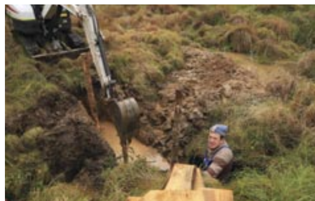
Fig. 68: It is practically impossible to install woody dams at high water levels so that they work well, Vchynice-Tetov location, September 2022 (I. Buřková)
