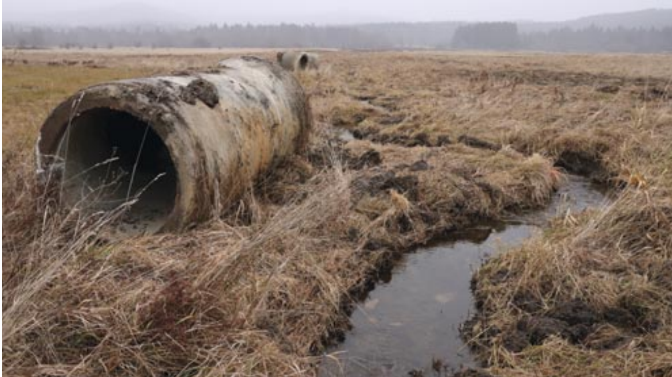
Fig. 82: Removal of concrete pipes forming the main drainage facility (HOZ) and restoration of the natural small stream at the Dobrovodské louky locality, immediately after restoration, November 2021 (I. Buřková)
