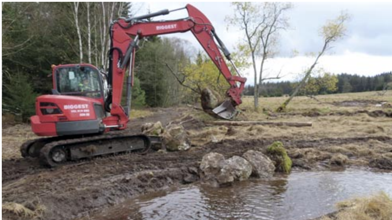
Fig. 142: Bringing the restored Kořenský stream out of the regulated channel in the Stráženská slat' locality. The downstream (in this case the left) bank of the stream, which runs along the reinforced dam in the canceled channel, was fortified with large boulders, February 2024 (I. Buřková)
