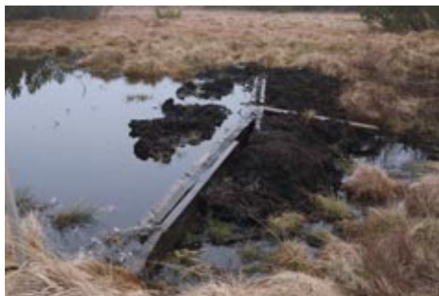
Fig. 105: Washing out unsprinkled and poorly inserted dams (I. Buřková)
