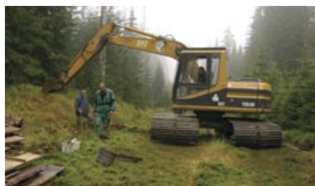
Fig. 72: Mud excavator with wide belts during the blocking of huge erosion grooves in the Černohorský močál mire, September 2014 (I. Buřková)
