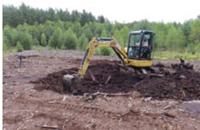
Fig. 89: Excavation of shallow depressions (pools) on the mined bog Vlčí jámy, August 2021 (E. Václavíková)
