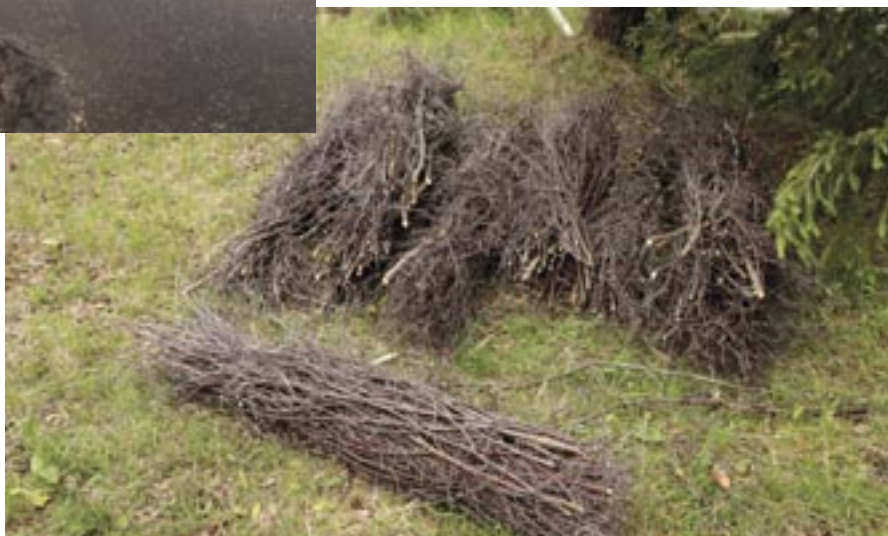
Fig. 107: Pontoon plates for increasing the bearing capacity of the terrain, Nové Údolí, November 2020 (I. Buřková)
