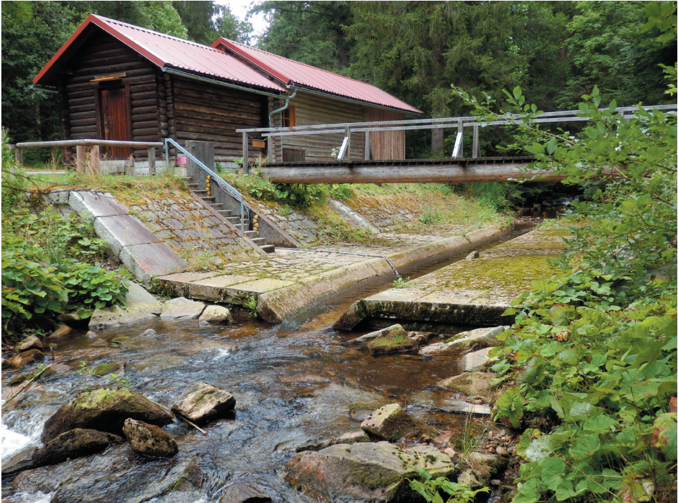
Fig. 2. The Taferlruck stream gauge (48°56'17.99" N, 13°24'45.13" E) with a cross section designed for low and high flow measurements (photo: W. Breit, 2015). Independent discharge measurement with a current meter is performed using the wooden bridge. Note that, up to now, the instantaneous flow varied between 0.09 and 24 m 3 .s -1 . In 2010, the downstream channel underwent reconstruction to reduce its barrier effect on fish migration.
